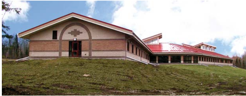
Construction of the ATEC Centre is now complete and should open in January once all equipment and furnishings have been installed.
