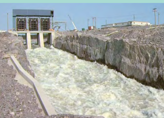
Above: Closure of the Taskinigup Falls – diverting the flow of water through the spillway.
