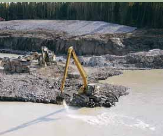
(Above and Below) Downstream cofferdam removal following completion of main dam.
