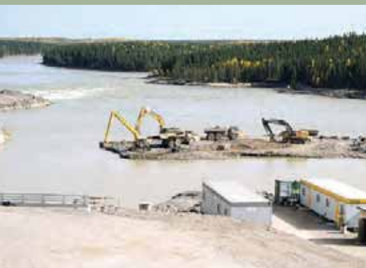
(Above and Below) Downstream cofferdam removal following completion of main dam.
