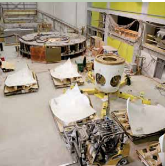
Turbine parts awaiting assembly in powerhouse.
