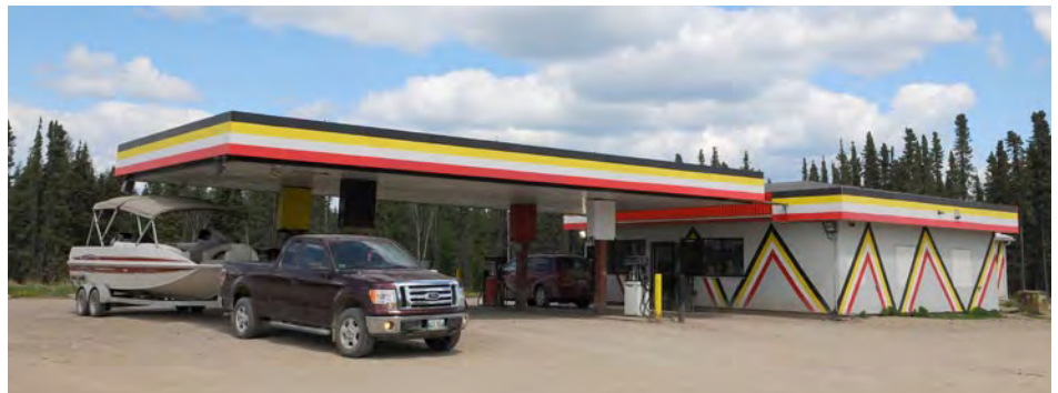
OT Gas Bar demonstrates the company's ongoing success and better meets the needs of customers.
